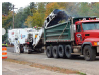
Milling of the surface layer
