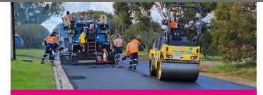
From here, the process was very simple, nothing else was required to be altered by FH, from mixing time, transportation, paving, raking and compaction. Speaking to the operators on the day, they advised that if we hadn't told them of the fibres, they wouldn't have known they were in there!
