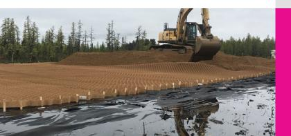
Case studies: (a) Neoloy-reinforced access road on existing saturated peat bog soil (CBR 1%) for MEG Energy, Canada; (b) High speed track stabilisation, Amtrak, US Federal.
